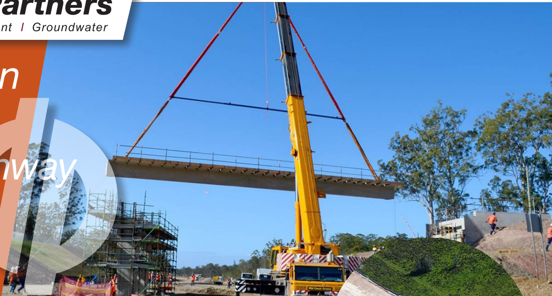
Bridge deck installation
