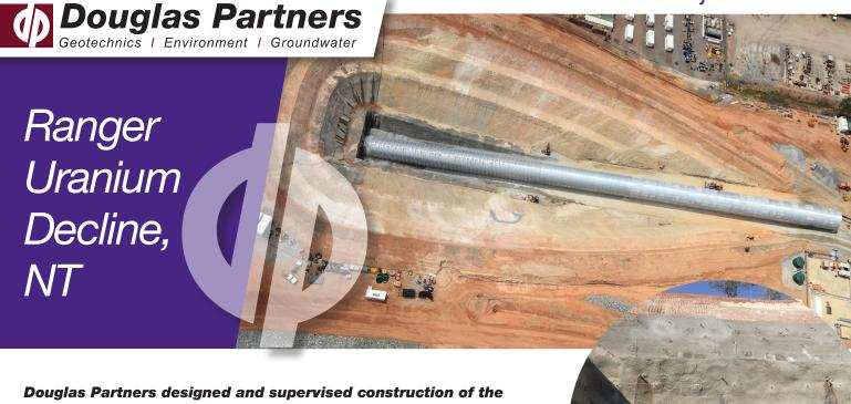
Douglas Partners designed and supervised construction of the Ranger Uranium box cut, tunnel portal and decline. The decline was 2220m long, 6m high by 5.5m wide. Initially Douglas Partners was asked to re-design the tunnel portal, previously designed by others. The re-design required a site investigation and re-design of the box cut.
