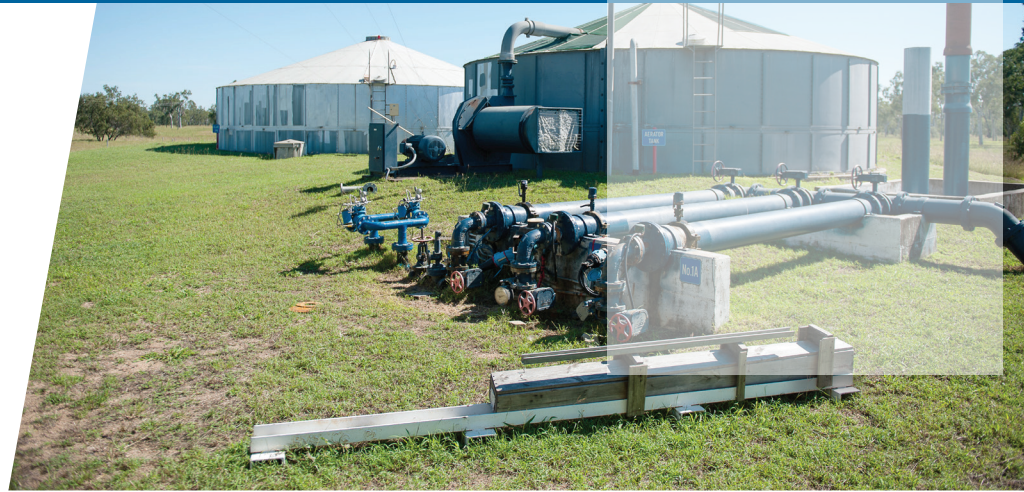
Braeside borefield comprises 16 production bores and provides ~3,000 ML/a of water to a number of coal mining operations, towns and rural properties in the Northern Bowen Basin
