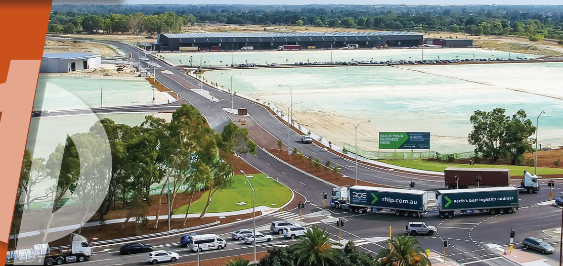
Roe Highway Logistics Park – Stage 1
