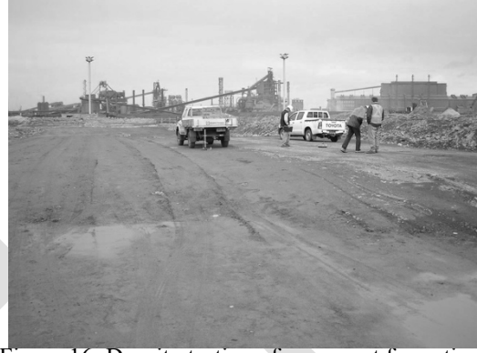
Figure 16: Density testing of pavement formation
