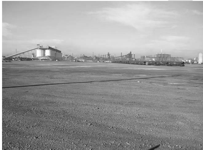
Figure 4: Hardstand area. Grain terminal to left and Steelworks in background.
