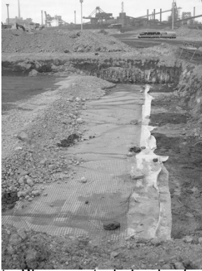
Figure 15: Placement of slag bridging layer
