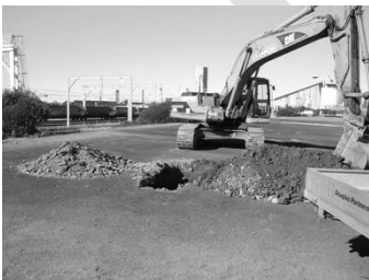
Figure 5: Test pit excavation
