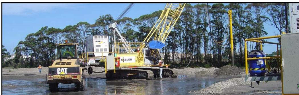
Figure 2: Installation of Stone Columns
