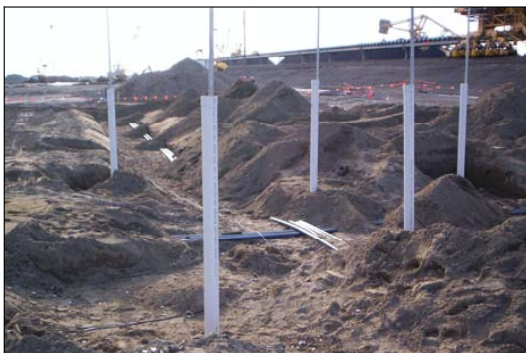
Figure 4: Instruments prior to placing fill
