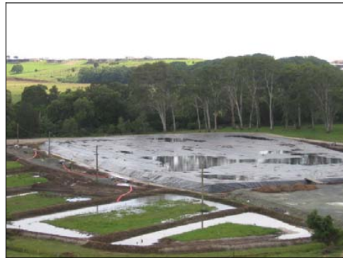
Fig. 5 - Vacuum consolidation (membrane system) in progress at Ballina (NSW)
