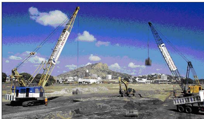
Fig. 7 - DR construction in Townsville (QLD)
